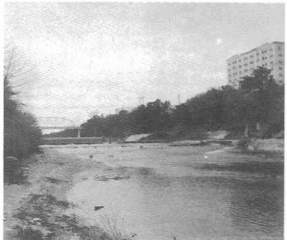
A. and B. The Guadalupe River channel at Kerrville, below dam (site 64). The channel bed is composed of extensively honeycombed dolomitic limestone beds in the upper member, Glen Rose Limestone. These porous and permeable beds facilitate considerable streamflow loss.
